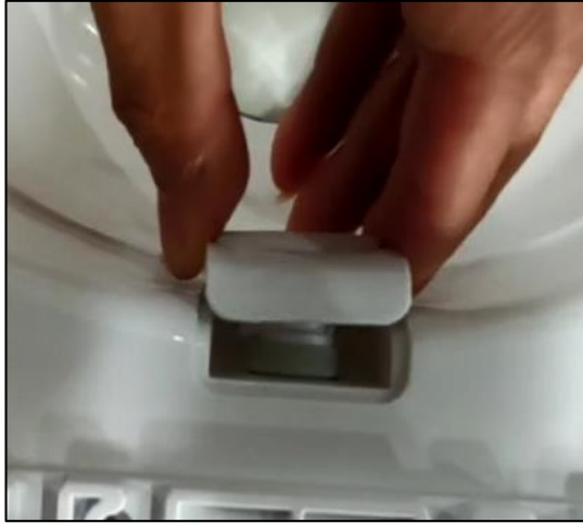
Step 1: Align the new nozzle with the outlet hole.
