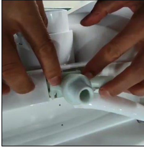
Step 1: Place the new inlet valve kit into the groove of the toilet base and press it flat
