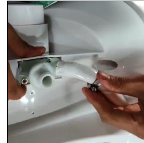
Step 3: Put the outlet hose back
