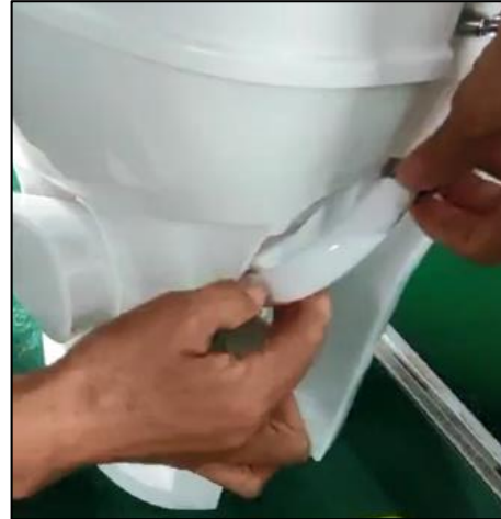
Step 2: Move the loosened hose clamp upward along the outlet hose
