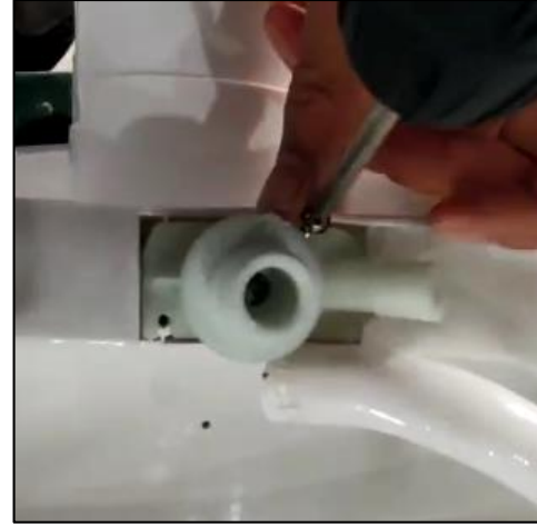
Step 2: Use a cross-head electric hand drill to tighten the fixing screws (torque 6~8KG)
