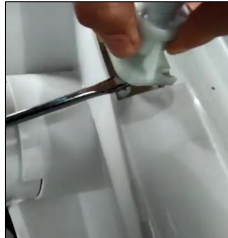
Step 5: Use a flat-blade screwdriver, insert it into the left bottom side of the inlet valve kit, and pry open the inlet valve kit
