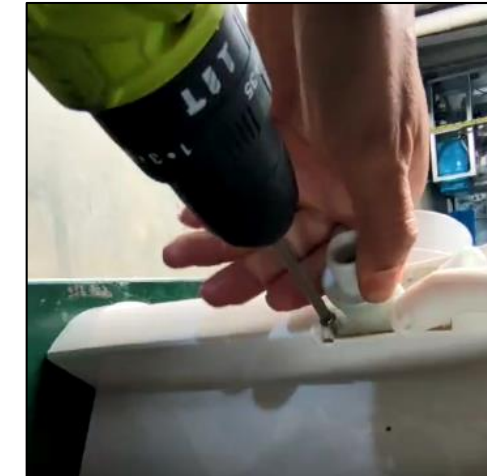
Step 4: Use a cross-head electric hand drill to loosen the 2 fixing screws of the inlet valve kit.
